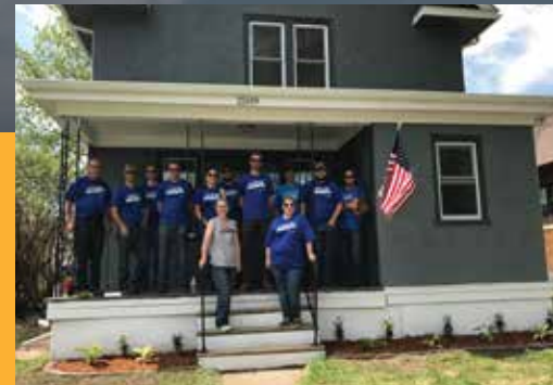
Employees from Minnesota Power and Delta Air Lines volunteered to work on the United for Veterans transitional house in May of 2018.
